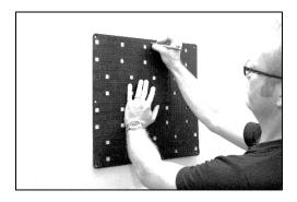
Step 3. Drill the 5 holes and insert wall plug
