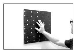
Step 2. Mark the 4 corners, and the top hole with a pencil (5 in total)
